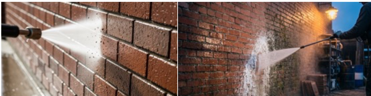
Figure 9: To clean red brick safely, use 500 to 1,500 PSI (pounds per square inch) with a wide-angle nozzle (25°–40°), ensuring the tip stays at least 12 inches from the surface to avoid damaging the mortar. For older or delicate brick, use even lower pressure or a soft-wash method. A pressure washer nozzle is designed to send powerful jets of water to clean surfaces, sometimes with the unintended consequence of damaging inside concrete or brickwork. This uses a nozzle creating cone-shaped sprays for highly directed water into specific areas. The nozzle type can be from almost 0° to as much as 40°, and this will allow different pressure levels striking a surface.
