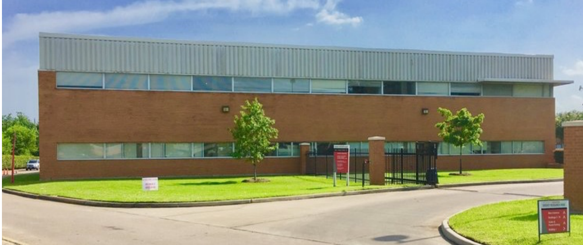
Figure 13: Building 2 at the Technology Bridge at the University of Houston after 7 years of exposure to freeze (20°F) to heat (105°F) with humidity levels of >95%, surviving 2 hurricanes.
