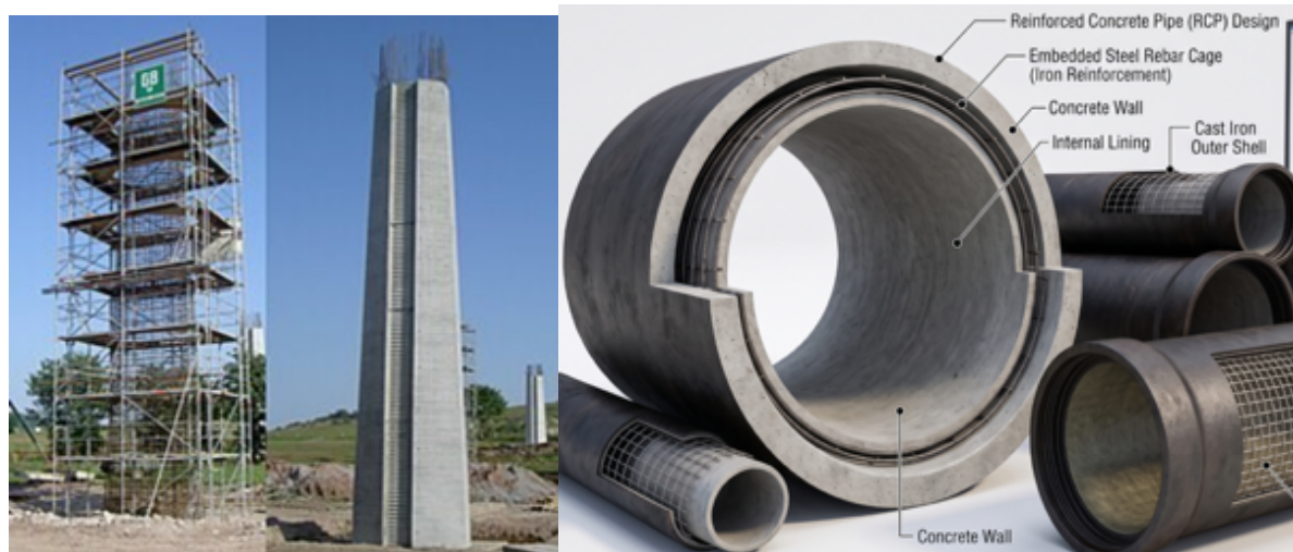
Figure 13. a) heavy, reinforced concrete column, seen before and after the concrete has been cast in place around its rebar frame. Photos: Benutzer:Störfix. Combination: Florian.Arnd, CC BY-SA 3.0 < http://creativecommons.org/licenses/by-sa/3.0/ >, via Wikimedia Commons, b) Structure of reinforced concrete pipe showing the concrete wall, inner lining, and embedded steel reinforcement susceptible to corrosion.
