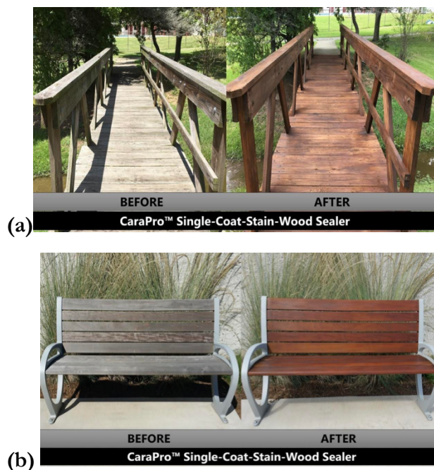
Fig. 9. Before and after comparison of Single-Coat-Stain-Wood Sealer (SCHN) application on outdoor wooden structures. (a) Public footbridge prior to treatment (left) and after SCHN application (right). (b) Park bench before (left) and after SCHN application (right).
