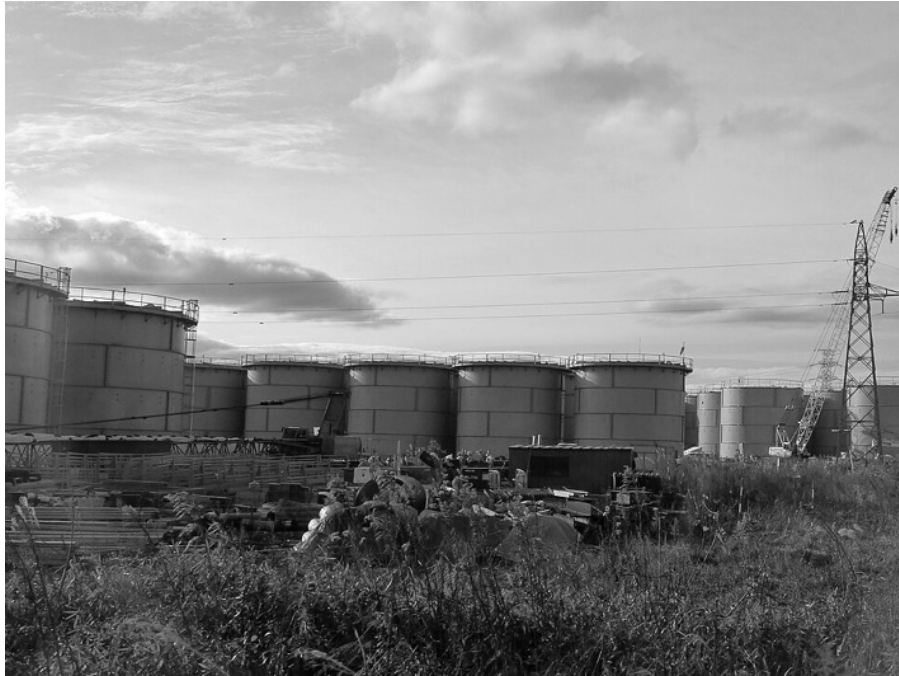
Figure 3 Storage tanks containing treated and contaminated water at the Fukushima Daiichi Nuclear Power Plant, December 2012. (Photo: IAEA / Gill Tudor, public domain)
